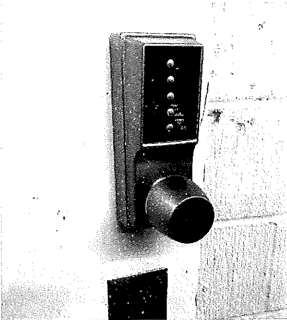
Photo 5 : Punch code lock on door to area with limiter
